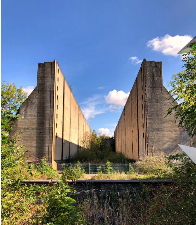
to bridge the height difference of 22 meters between Saale und Saale-Elster Canal
