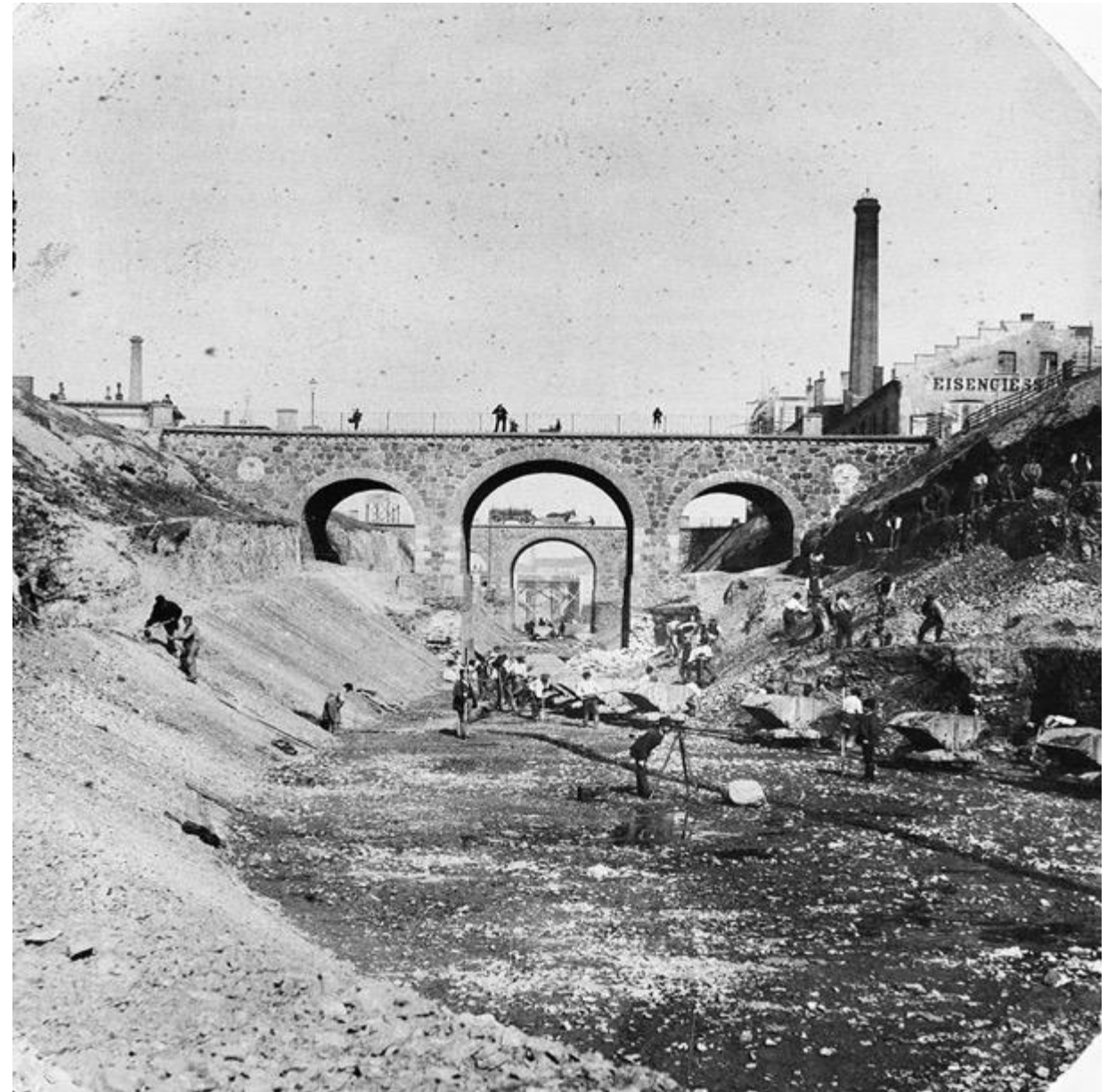
Building the canal: construction work 1885
