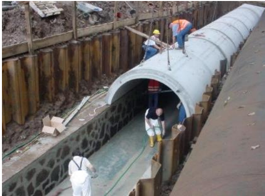
Renovation of sewer system
